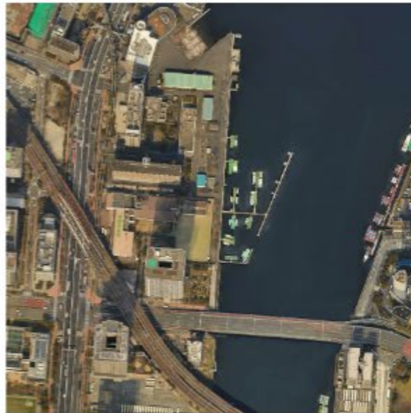
(b) Cross-river bridge.
